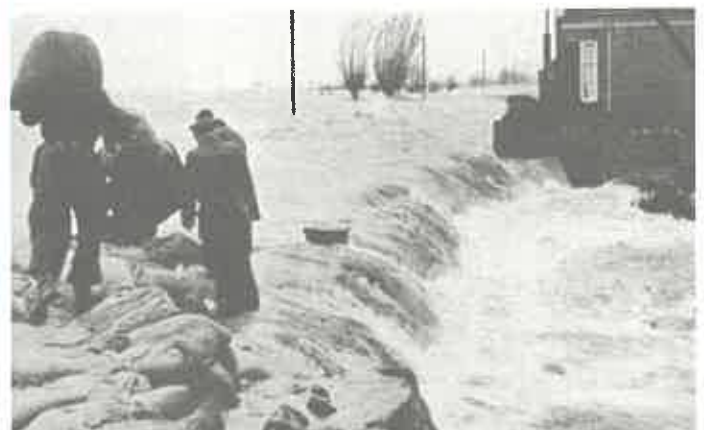
fig. 23 Breached dyke in February 1953
